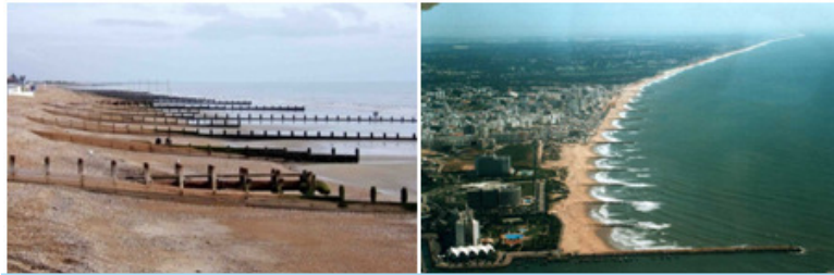
Fig.8. 18: Groins built for trapping long shore currents
