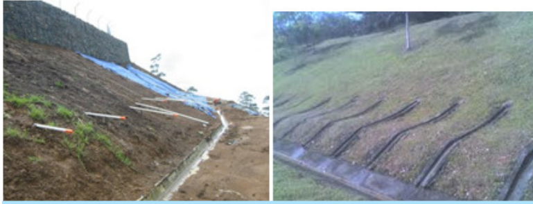
Fig. 8.13: Drainage pipes along slopes.
