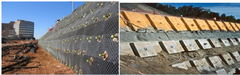
Fig. 8.12 :Rock bolts to prevent slope failure
