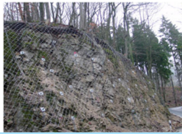
Fig.8.11: A slope covered with wiremesh
